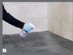
Before the final washing stage, PCI Durapox® Finish (liquid) is sprayed onto the surface after about 60 minutes. Alternatively, PCI Durapox® Finish (concentrate) can be added directly to the washing water.
