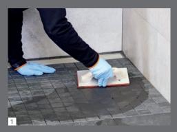
Very easy grouting without residues using PCI Durapox® Premium. The product is very easy to process using standard tools. No special epoxy resin tools are needed. After about 10 to 45 minutes, the grouted surface should be worked over with a sponge float and then washed down cleanly.
