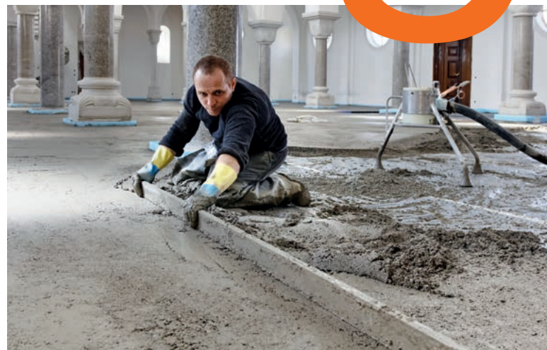
Screeds laid using PCI Novoment® Z1 can already be walked on after about 3 hours and covered with ceramic tiles after about 1 day.
