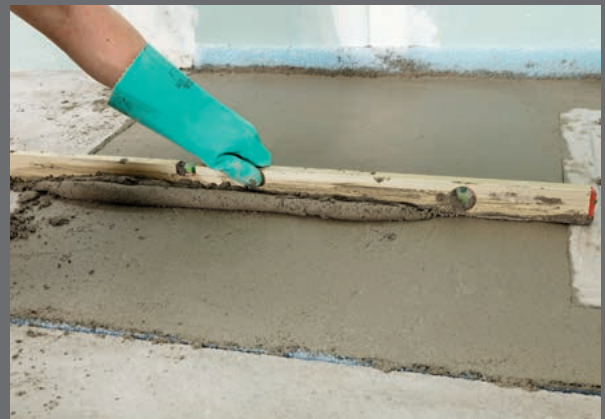
PCI Novoment® Light allows layer thicknesses from 20 to 80 mm and is insensitive to moisture – ideal for the use in permanently wet areas and sloped surfaces.
