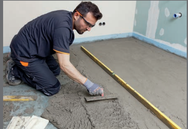
Additional smoothing of the surface is hardly necessary after stripping and rubbing.
