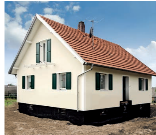
Waterproofing with polymer-modified thick bituminous coatings
